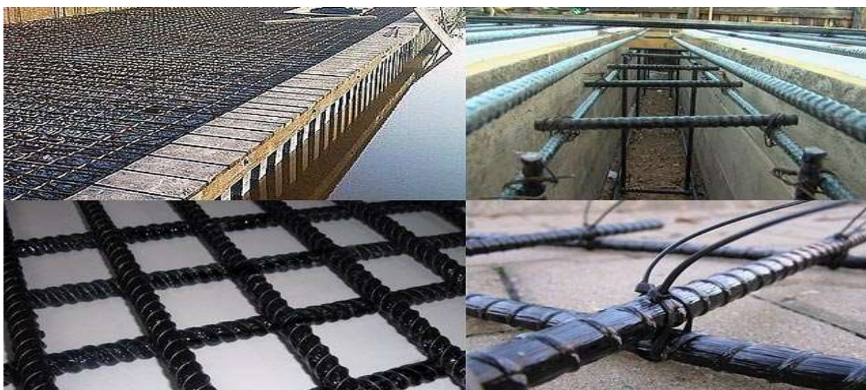
The use of basalt-plastic reinforcement in construction.
